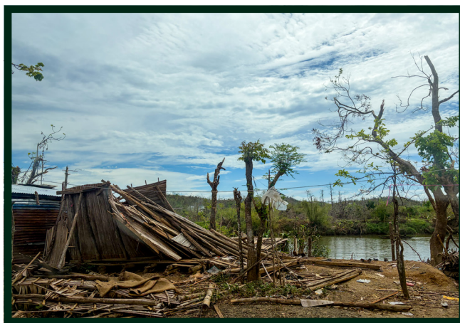
A ShelterBox team is in Madagascar together with our partner Welthungerhilfe, conducting damage assessments and holding focus groups with local people to better understand the needs of the communities that have been affected.
