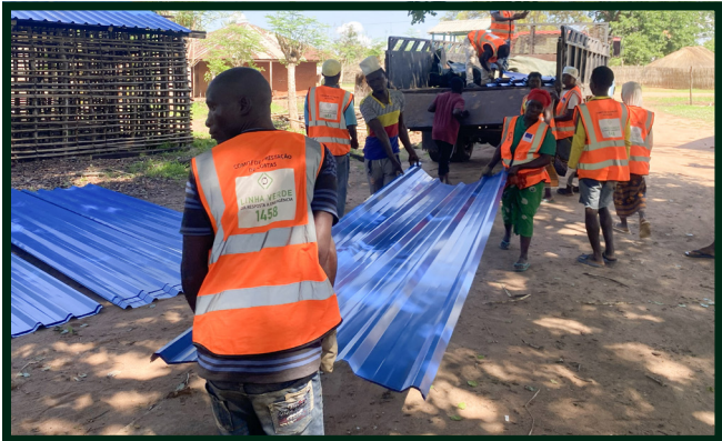
Through an ECHO-funded conflict response in Cabo Delgado (Project 3), with CARE Mozambique and others, we supported displaced communities with 500 transitional shelters (timber frames and tarpaulin or corrugated iron roofs).
